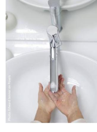
after going to the toilet, for example, or for rinsing out a coffee cup at the sink. The water is drawn off for such a short time that there is often no hot water at all. In the middle position, however, the hot water inlet also opens and the hot water meter turns on for no reason. In reality, we don't use any hot water at all at such times, but we pay for the hot water to flow in the supply pipe only to cool down again. There's no reason not to wash our hands with cold water!
